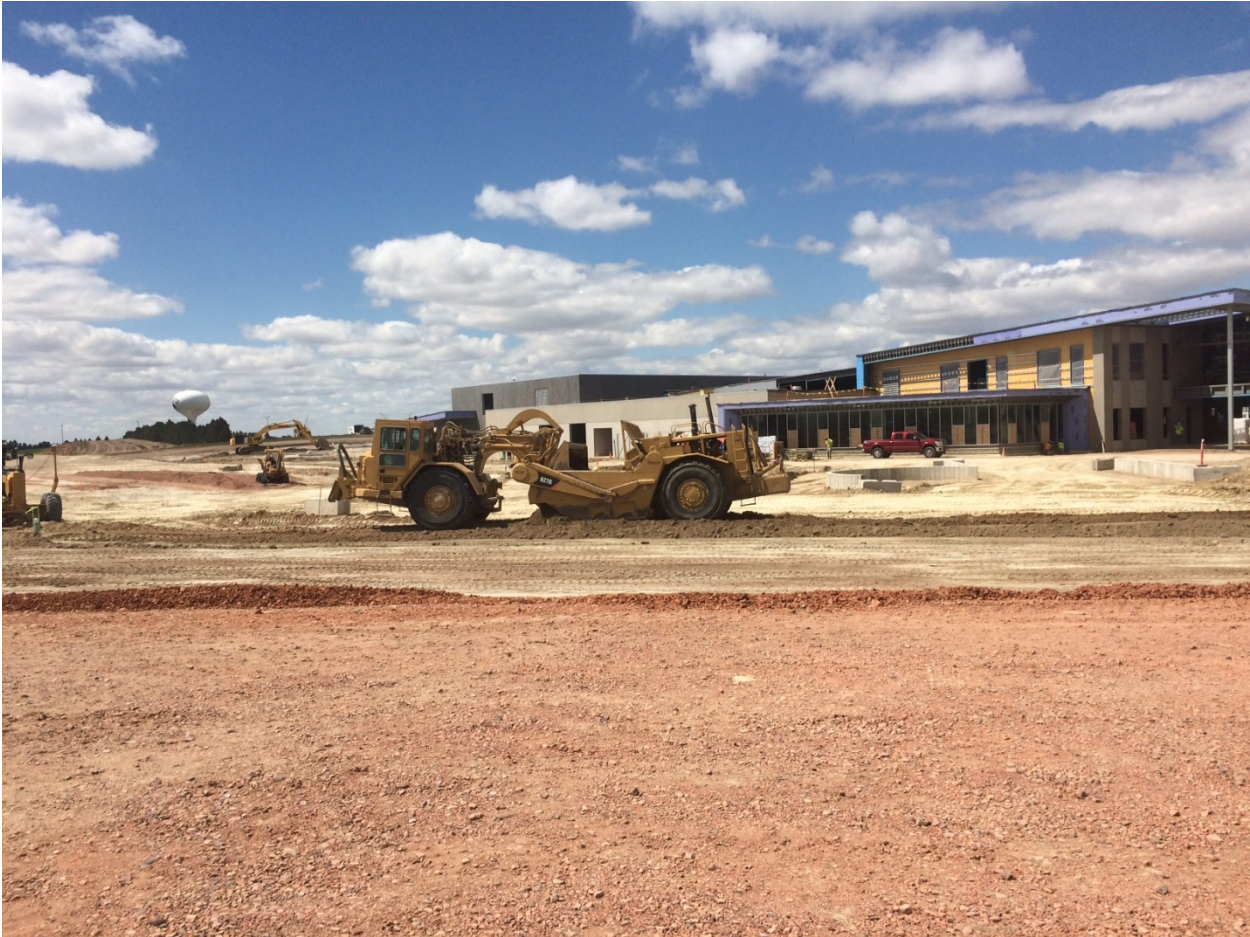
Front Parking Lot Grading
