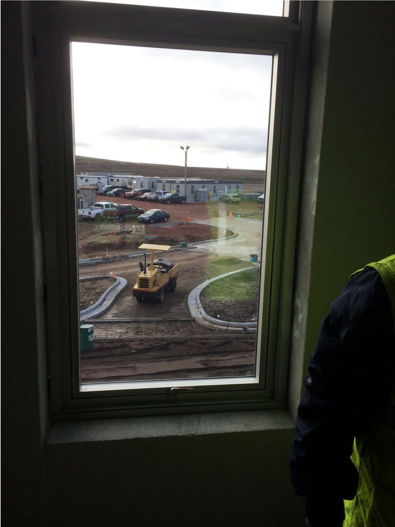
South window installed
